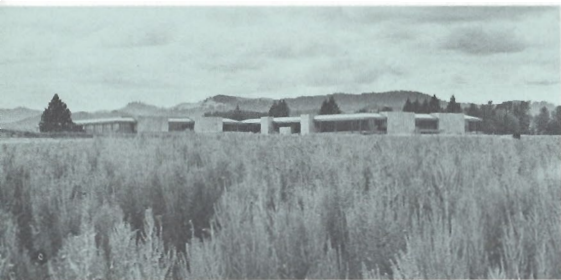
Field frames HP plant.
